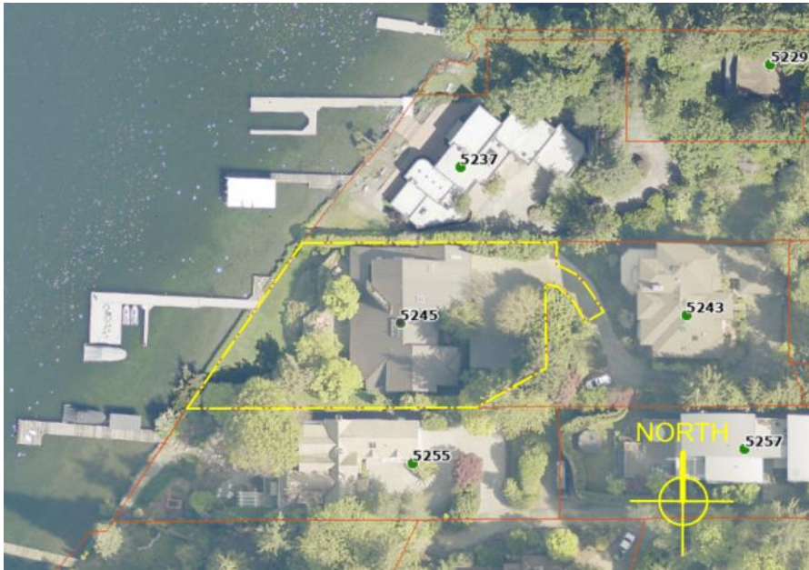
Plate 1: Aerial view of the site.
