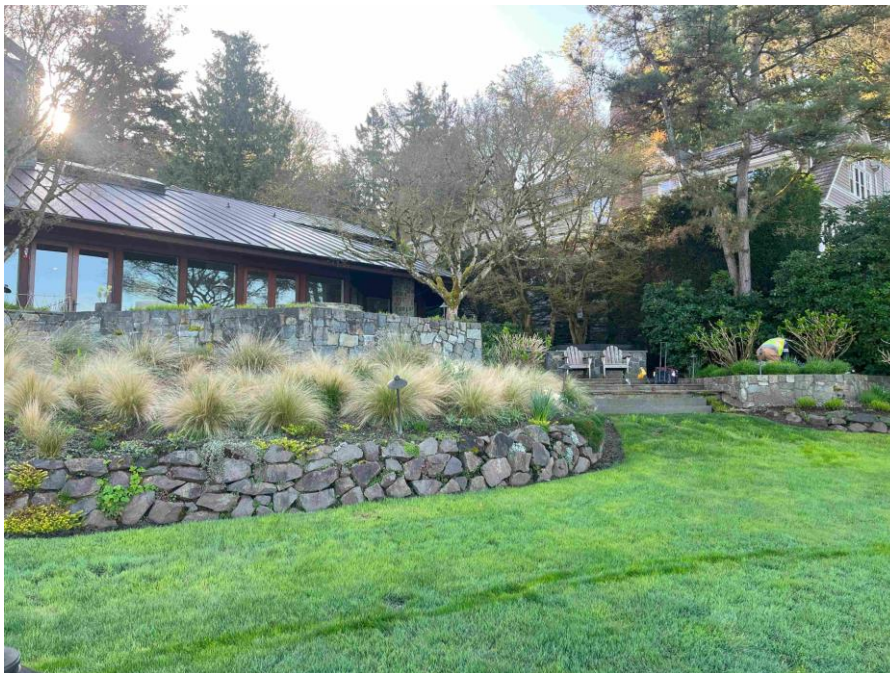
Plate 2: Rear view of the existing residence. Looking southeast from the west property line in the approximate area of the proposed sauna.
